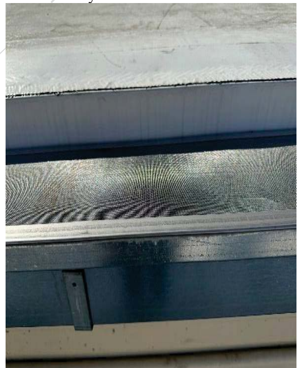
Gymnasium – Micro-Mesh Gutter Guard
