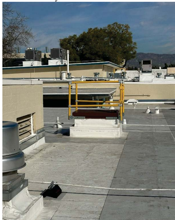
Gymnasium – Roof Hatch
